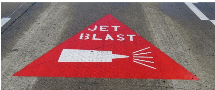
Figure 53. Marking indicating a risk of jet blast
