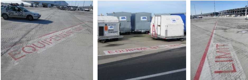
Figures 48, 49 and 50. Demarcation markings for equipment storage areas
