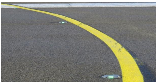
Figure 62. Balisage de taxiway
